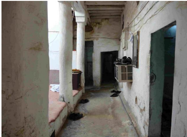
Fig. 4.33: Using plaster for covering the internal walls
