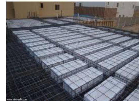
Fig. 4.54: Roof structure – reinforced concrete integrated with blocks
