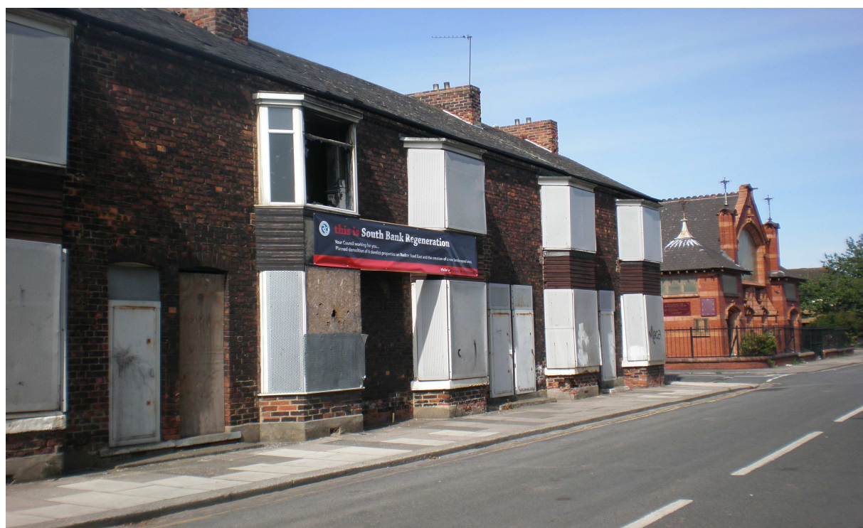
Figure 1: Boarded up housing in South Bank, 2011
