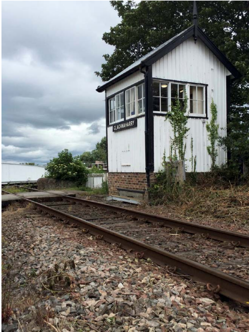
Figure 4: Clachnaharry Signal Box (1890). Only modern track and enclosure of the lead way (opening through the brick plinth) show any changes since construction. The open swing bridge is visible to the left.
