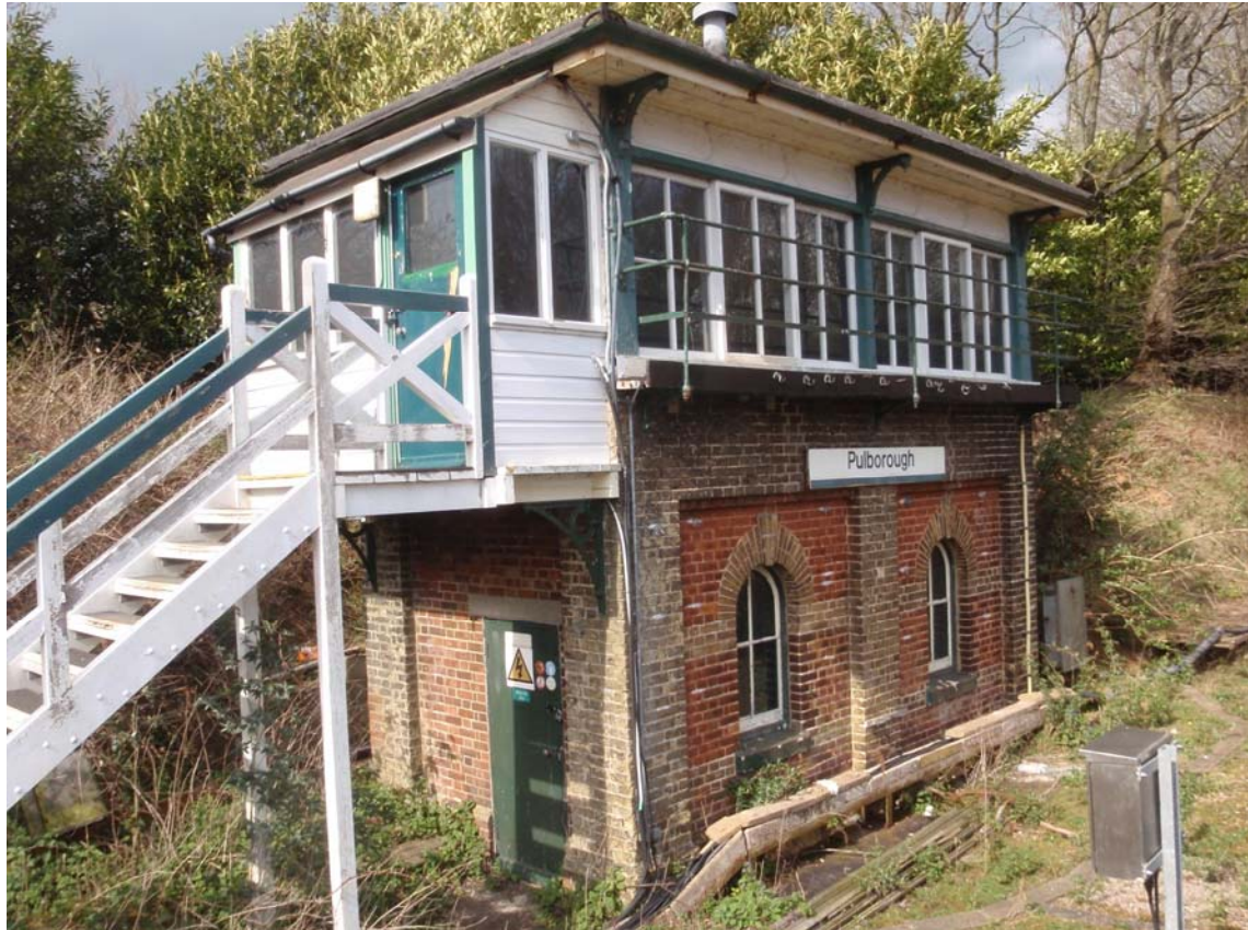
Figure 7: Pulborough Signal Box (1878). The London Brighton and South Coast Railway (LB&SCR) made extensive use of the standard modular signal box designs by the signalling manufacturer Saxby and Farmer (John Saxby being a former employee of the LB&SCR). Pulborough Signal Box is a Saxby and Farmer Type 5 design, although the unsympathetic porch is a later addition that pre-dates the listing. The staircase is a replacement.
