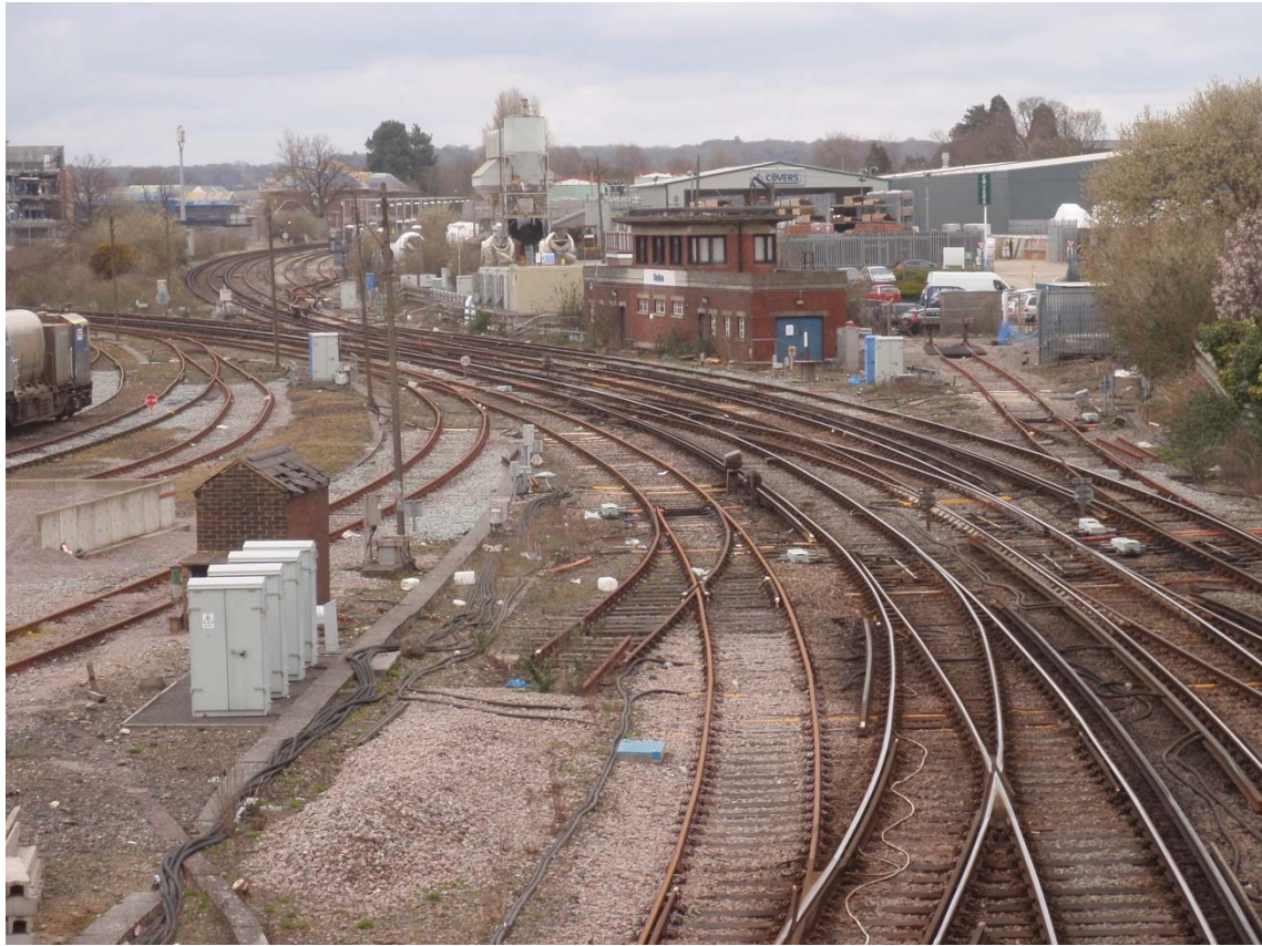
Figure 6: Horsham Signal Box (1938), being a Southern Railway type 13, an Art Deco influenced design known as the 'Odeon' style. Opposite the signal box is the original goods yard, now slightly reduced in size and in use for civil engineering trains. Behind the signal box was situated the former engine shed, redeveloped as industrial units. Recognisably a signal box and, other than the missing engine shed, the railway landscape is presumably recognisable in comparison with 1938.
