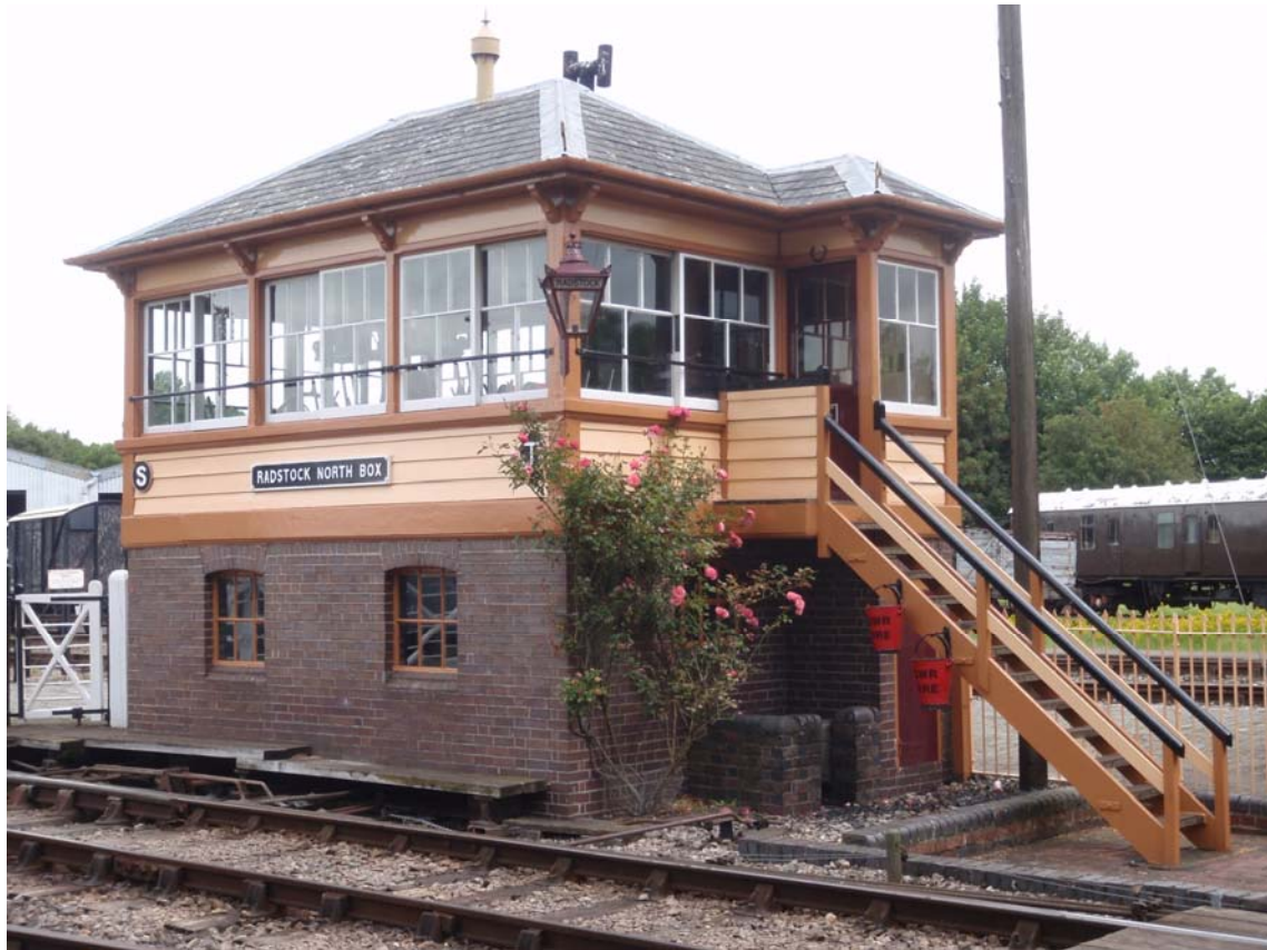
Figure 9: Radstock North Signal Box (1909). In an equivalent manner to Frome Mineral Junction Signal Box, this is a relocated operating level on a replica locking room plinth. An attempt is made to match the bricks to original, although again is apparently in contemporary bricks. Note the effort to provide a contextual interpretation in the relocated setting.
