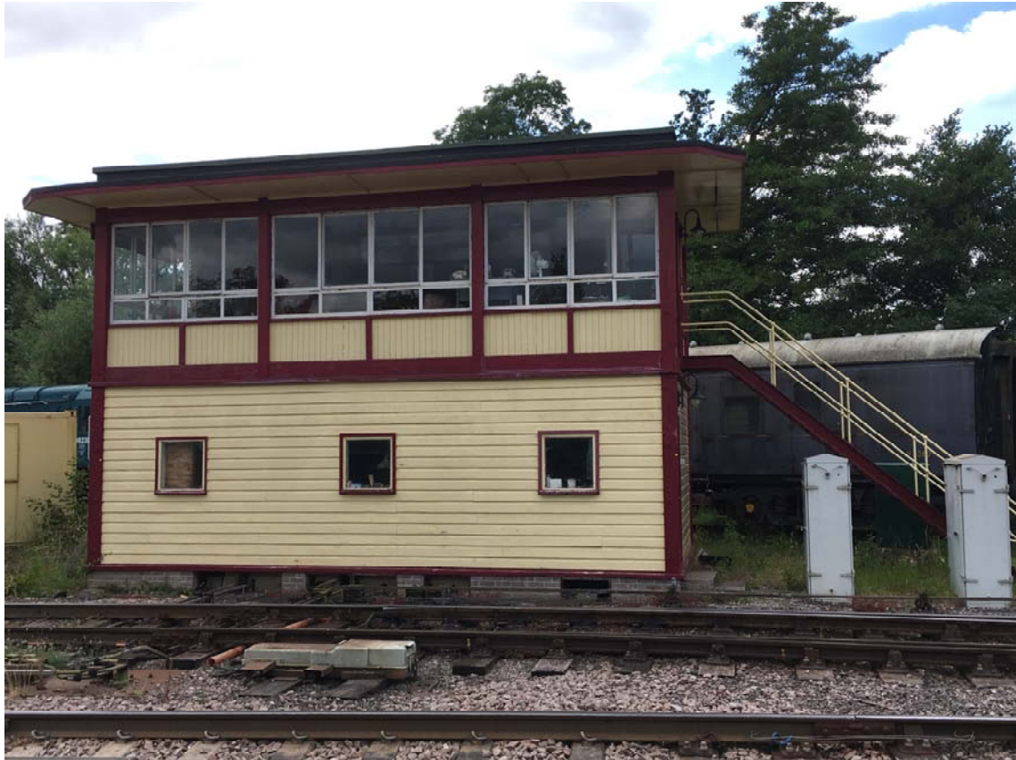
Figure 10: Lydney Junction Signal Box, formerly Heysham Harbour Signal Box (1970). Relocated in 1996, the entirely timber construction facilitating relocation, this well-presented signal box serves an operational requirement on a heritage railway.
