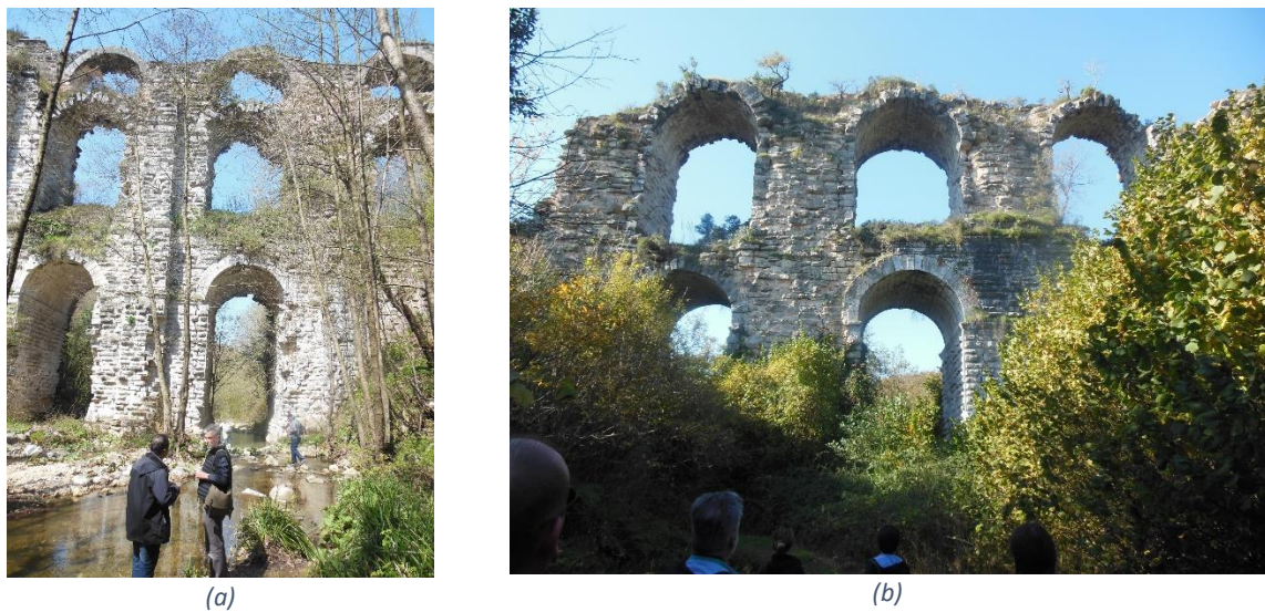
Figure 2: Aqueduct bridges at (a) Kurşunlugerme and (b) Kumarlıdere
