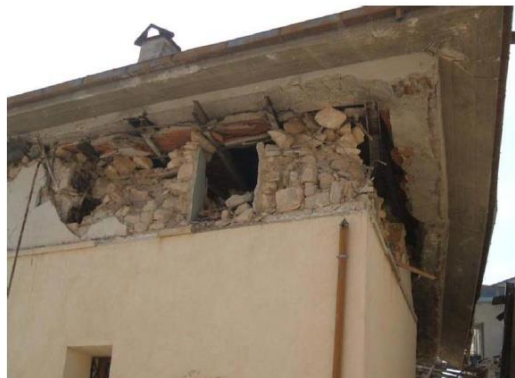
Figure 3. Effect of earthquakes on historic buildings where timber roof beams were replaced with RC elements.
