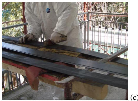
135 Figure 4. Different retrofitting methods using FRPs: (a) FRP sheets; (b) FRP pultruded elements at the 136 compression side; (c) CFRP laminae.
