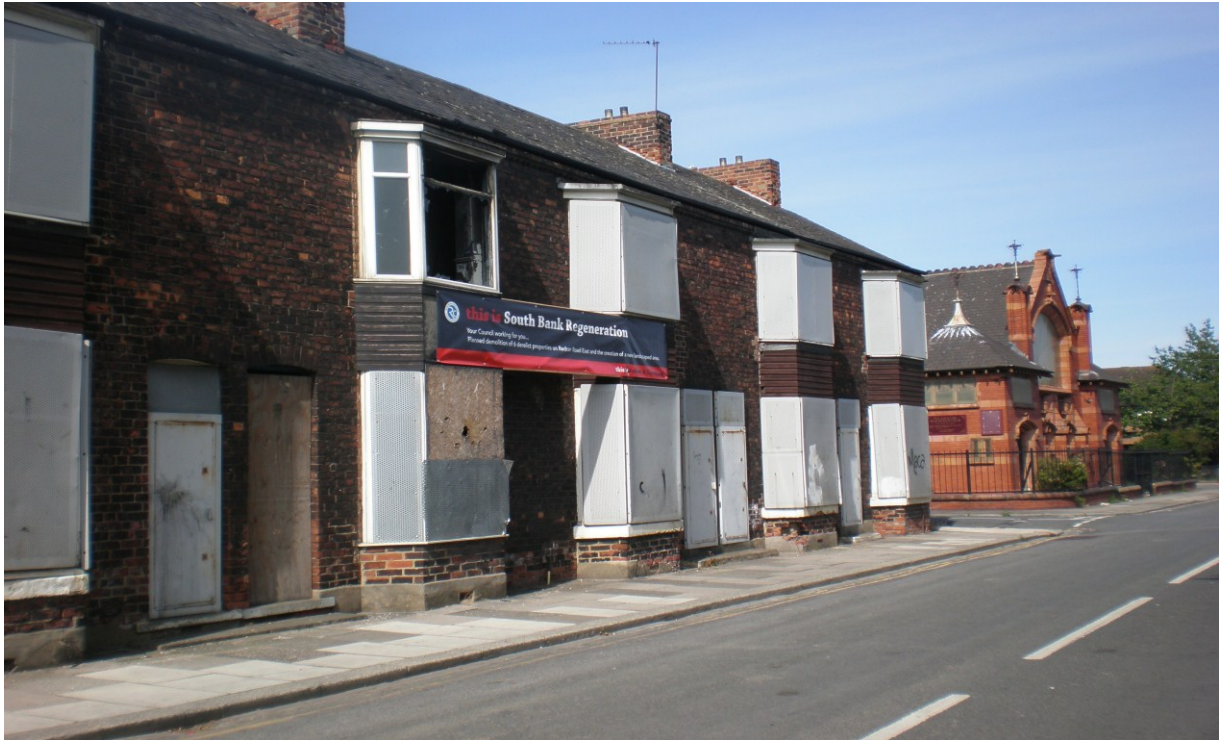
Figure 1: Boarded up housing in South Bank, 2011
