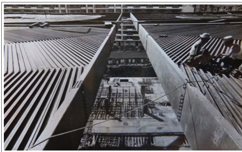
Figure 14: The Palace of Labour, the original roof in steel, removed in 1963. [Courtesy of PlannING]
