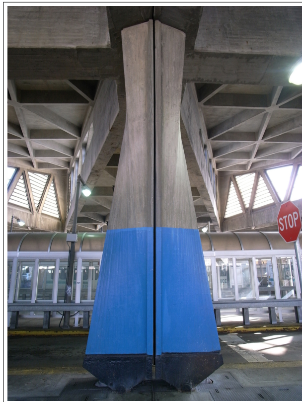
Figure 1: The double steel pin at the bottom of the central column. [MC]
