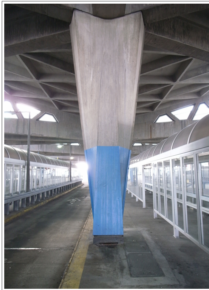
Figure 3: The variation in the profile of the central column. [MC]
