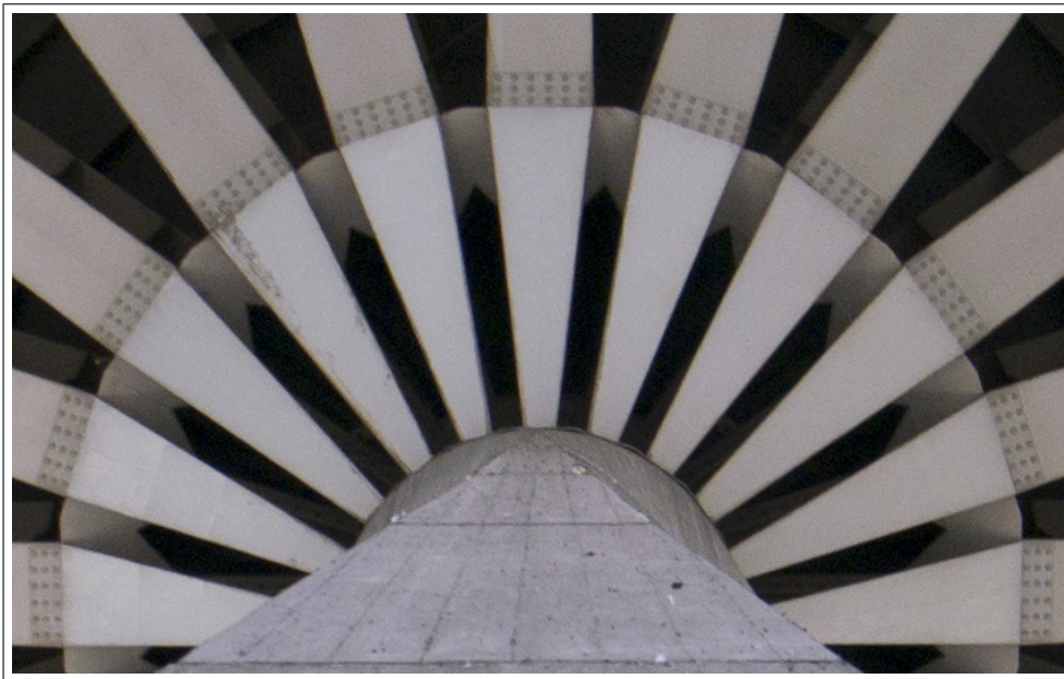
Figure 6: Detail of the bolted connection capital-beams. [MC]
