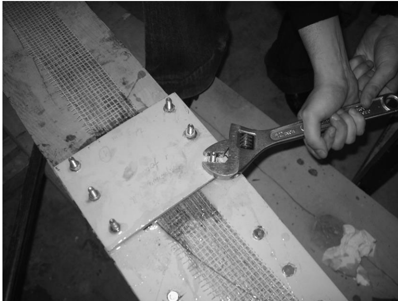
Figure 10. Prestressing technique: the clamp.
