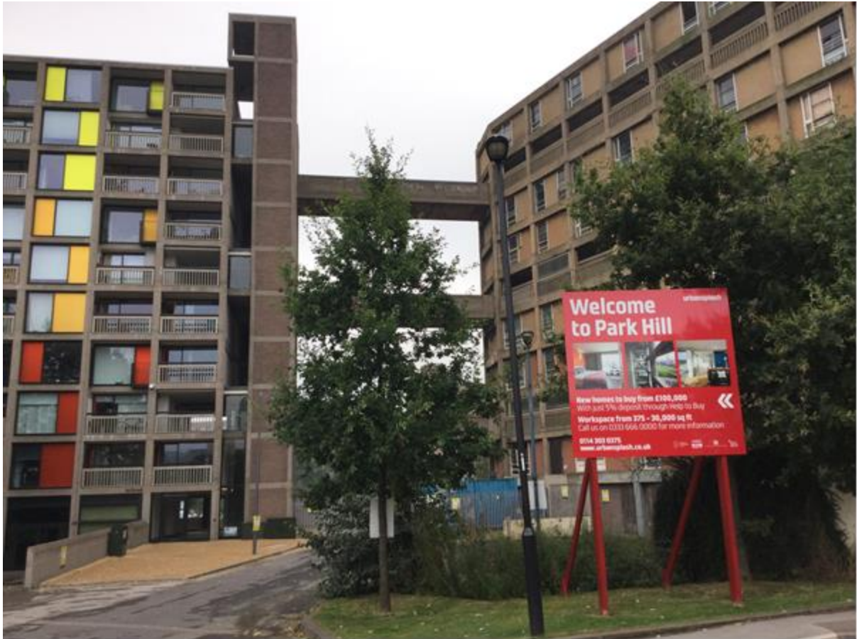
Figure 2: The Park Hill estate in Sheffield, 2016: a renovated block (on the left) adjoined to an evacuated block awaiting renovation (on the right)
