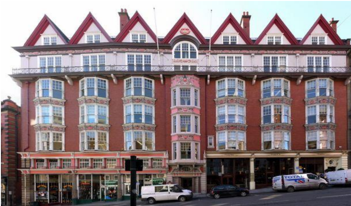
Figure 2.3 Cathedral Buildings, Newcastle upon-Tyne
