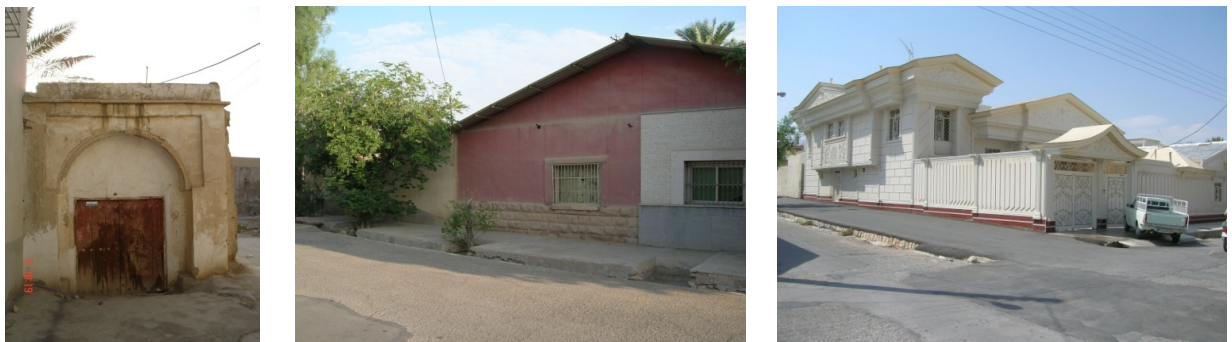
Figure 1: Pre-Earthquake (Left), Post-Earthquake (Middle) and Transformed (Right) façades in Lar.
