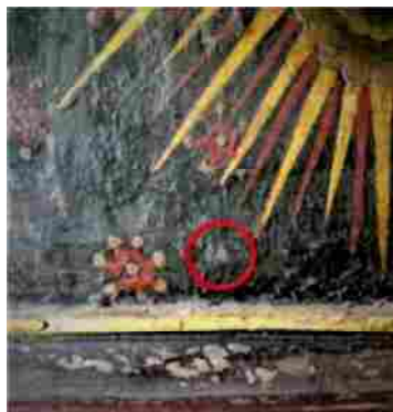
Fig 4 Showing sample area and flaking paint wear
