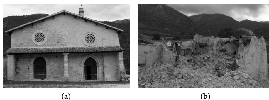
Figure 12. St. Savior's, near Norcia, Italy: Before (a) and after (b) the quake.
