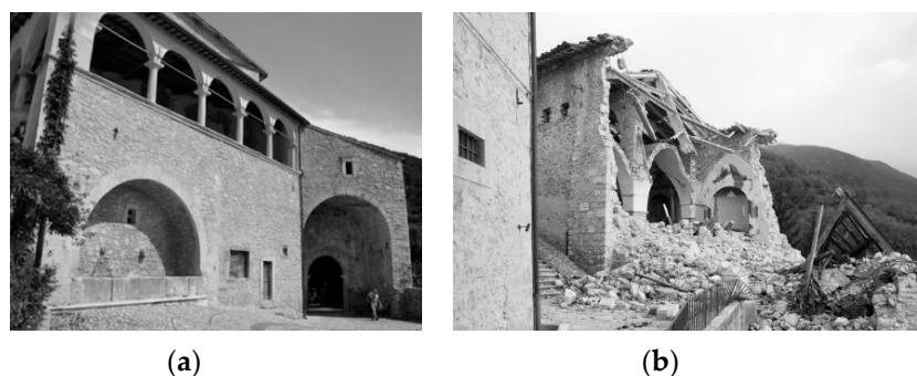
Figure 13. St. Andrew's in Campi, Norcia, Italy: Before (a) and after the quake (b).
