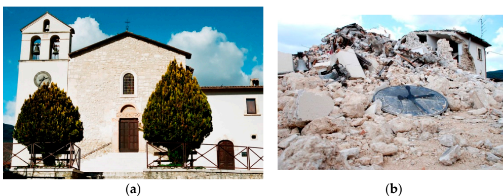
Figure 5. Parish Church of Tempera, near L’Aquila, before (a) and after (b) the 2009 quake: Replacement of timber-beam roof and grout injections were used to reinforce this historic construction in 1984.
