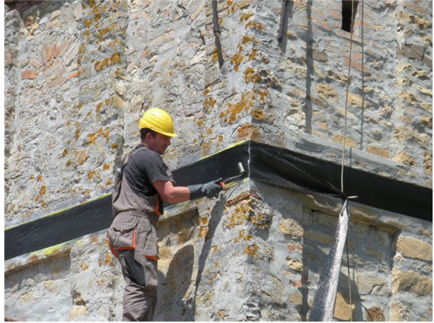
Fig. 2 Example of an “innovative” retrofitting solution using FRP unidirectional strip
