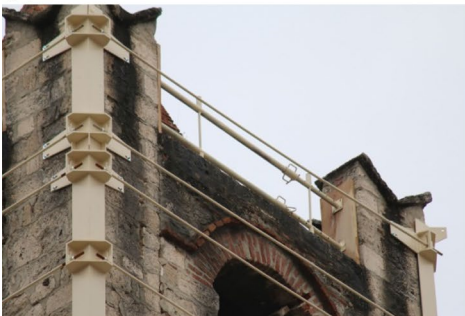
Fig. 3 a Traditional wrapping of a bell tower using steel bars, b application of unidirectional SRG strip
