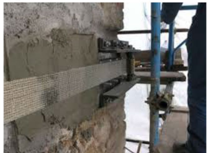
Fig. 3 a Traditional wrapping of a bell tower using steel bars, b application of unidirectional SRG strip
