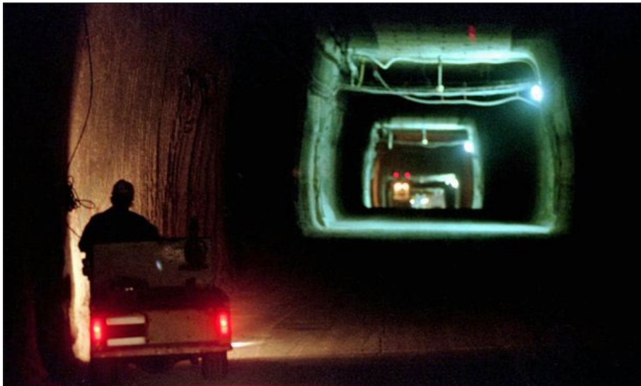
Construction of the Waste Isolation Pilot Plant in New Mexico, an underground nuclear waste dump. Photograph: Eric Draper / AP.
