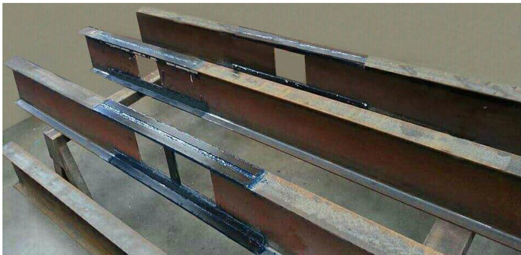
(b) Upturned specimens during curing of adhesive
