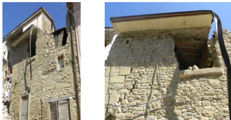
Figure 10. A building in Accumoli, near Rieti, in Italy: a large number of large cut stones was used here. This highly increased the level of connection between the wall leaves (combination No. 7, Table 5: cut stone masonry, medium-quality mortar, and effective connection between wall's leaves). For the upper part of this building, the quality of the masonry is lower and the wall leaves seem unconnected (combination No. 5, Table 5: cut stone masonry, medium-quality mortar, and non-effective connection between wall's leaves). The masonry of the upper part of this building disaggregated during the 2016 Central Italy earthquake.
