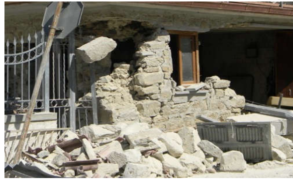
Figure 11. Pescara del Tronto, near Ascoli Piceno, in Italy. This is an example of cut-stone masonry, very weak mortar, unconnected wall's leaves (Combination No.2, Table 6). The building failed due to masonry disaggregation.
