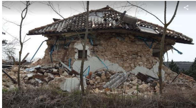
Figure 8. A collapsed building in Campi Basso, Norcia, Italy: The masonry (combination No. 1 of Table 4) of this building disaggregated during the earthquake.
