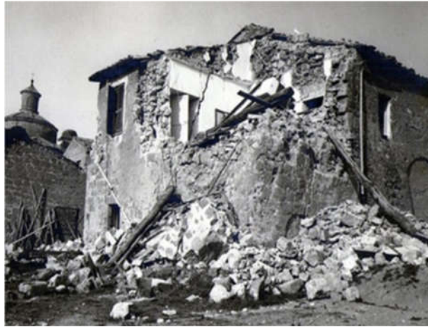
Figure 12. Tuff stone building in Tuscany, Italy, after the 1971 earthquake: the masonry typology can be classified in combination No. 1 of Table 7: irregular stones, non-horizontal bed joints, unconnected wall leaves, and very weak mortar. The failure mode is by disaggregation.
