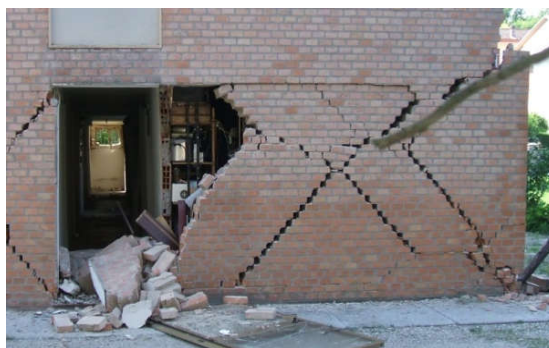
Figure 17. Failure mode of a building made of bricks and cement mortar (San Possidonio, Italy).
