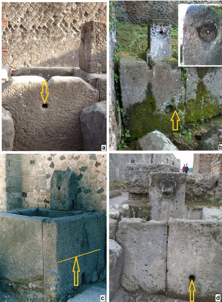
Fig. 12 Fountains presenting elements modified in ancient times. a Fountain 32 modified overflow with the piercing of a circular hole below the original channel, b Fountain 37 modified basin volume (bottom elevation) and reduction of the spout orifice, c Fountain 24 modified basin volume (bottom elevation), d Fountain 6 modified basin volume (bottom elevation)
