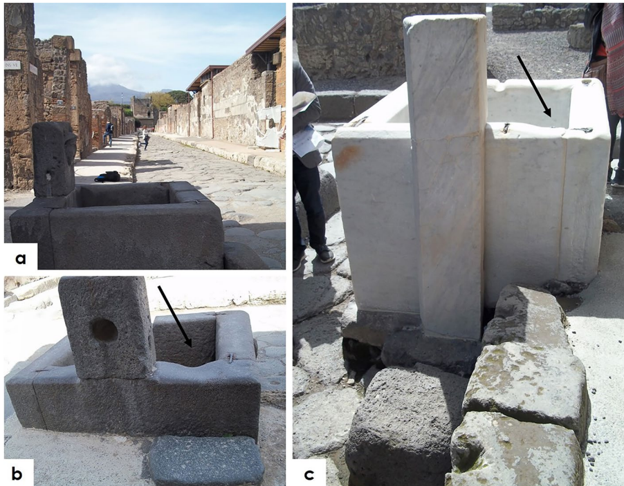
Fig. 4 a Example of the most common orientation of the fountains in Pompeii, with the spout stone on the side of the footpath and the overflow channel in front, b signs of wear near the spout stone due to the basin being accessed from the footpath, c example of a fountain with the stone spout located perpendicularly to the footpath, showing signs of wear on the footpath side
