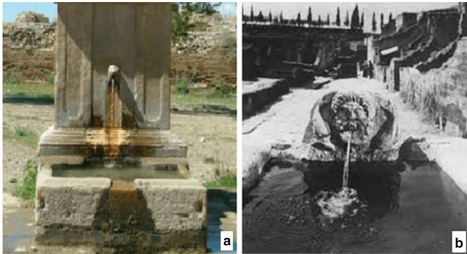
Fig. 14 Example of overflowing lacus supplied with a flowrate close to the minimum average discharge calculated for Pompeii fountains. a Timgad (courtesy of El-hadi Tebbane, flickr public collection), b Herculanum (Hartnett 2008)
