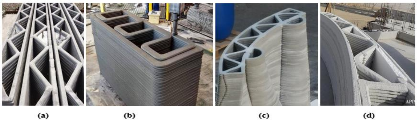
Figure 1. Examples of 3DPC wall panels with different cross-sectional arrangements: (a) triangular-shaped [25]; (b) lattice-shaped 3DPC wall by ETESIAS [26]; (c) sinusoidal-shaped 3DPC wall by Gosselin et al. [27]; (d) sinusoidal shaped, from the world's largest 3DPC building in Dubai [28].
