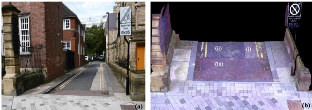
Figure 3.4. Field site: The field site was located adjacent to St James Church on Northumberland Road, Newcastle Upon Tyne, UK Grid Reference NZ 25112 64814. (a) Conventional photograph of the field site. (b) Point cloud panorama of the site captured using the Faro Focus 3D X Series phased-based laser scanner. The three surfacing materials studied are (i) surface dressing, (ii) dense bitumen macadam, and (iii) hot rolled asphalt.
