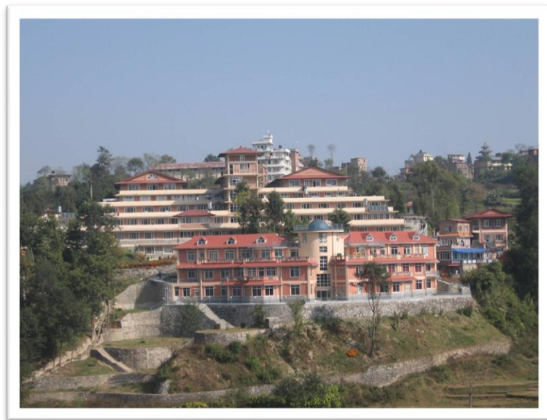
Figure 6.1: The ever expanding buildings of Dhulikhel Hospital
