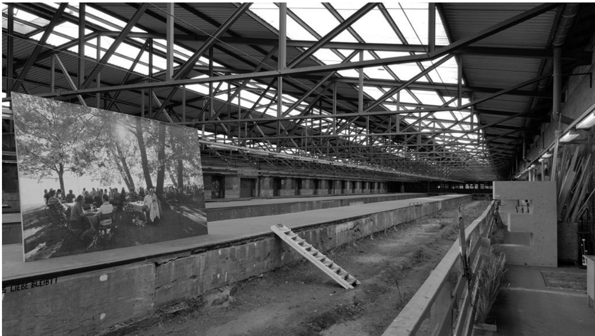
Figure 7.8 The central hall of the Oberhafen and its 4,000sqm. roof.
