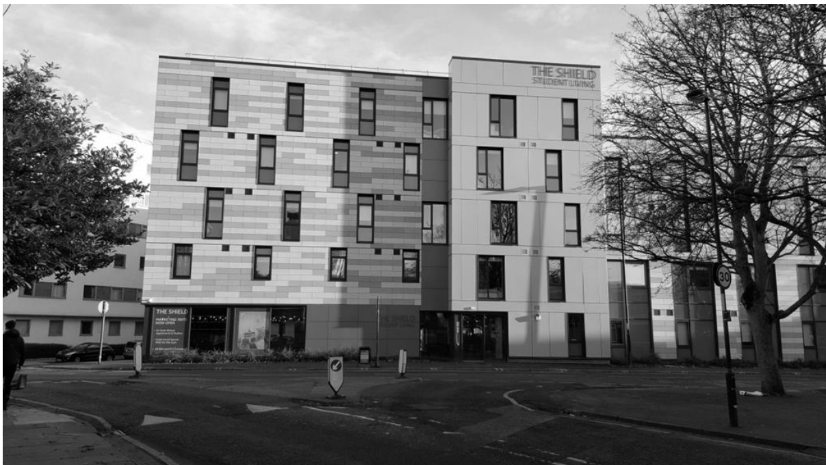
Figure 6.4 Student accommodation block on edges of Ouseburn.
