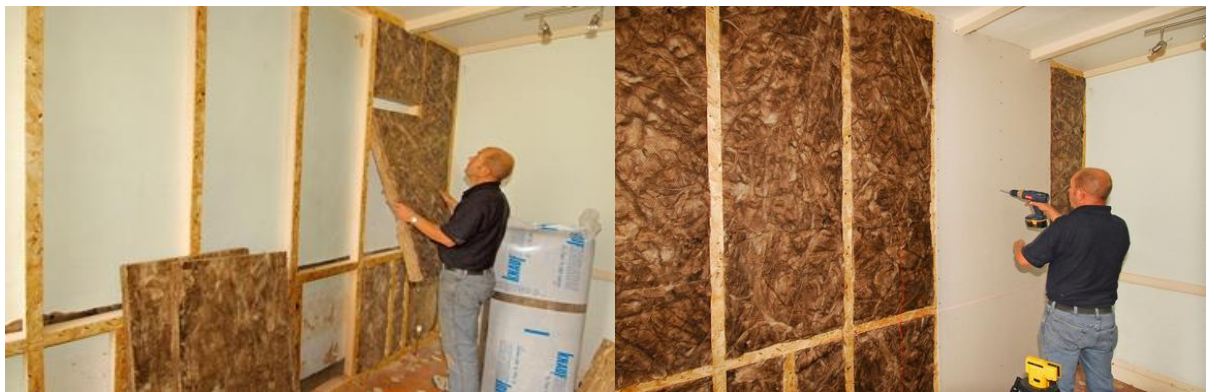
Figure 2.21 Internal solid wall insulation process (GREENAGE, 20016)
