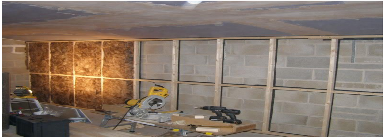
Figure 2.22 Back solid wall insulation process (GREENAGE, 2016)
