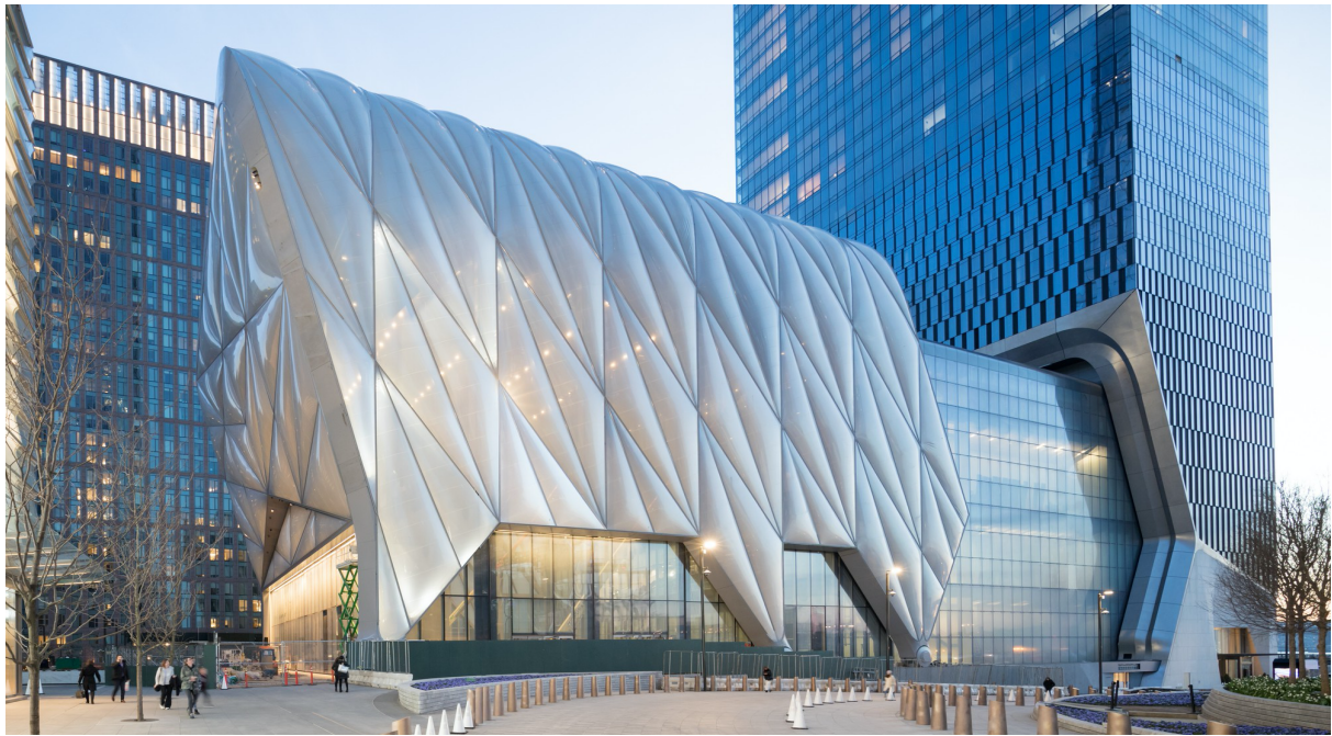
Figure 5. Moveable telescoping roof of The Shed, New York.
