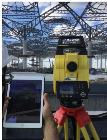
Fig. 6. Real-time progress monitoring and engineering surveying in IGA construction site
