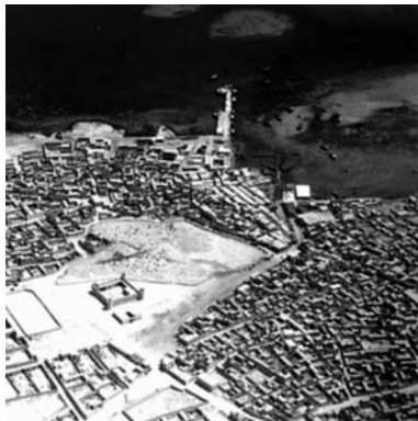
Figure 2b. The old urban fabric of Doha. Source: Msheireb Properties.
