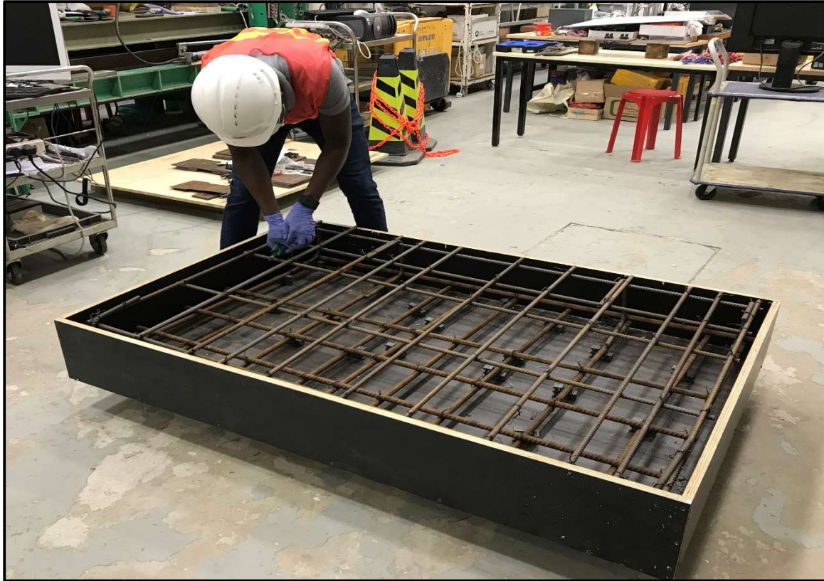
Fig. 3. A simulated manual rebar tying activity
