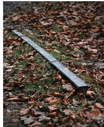
A surviving length of P&DR rail at Yelverton. Author
