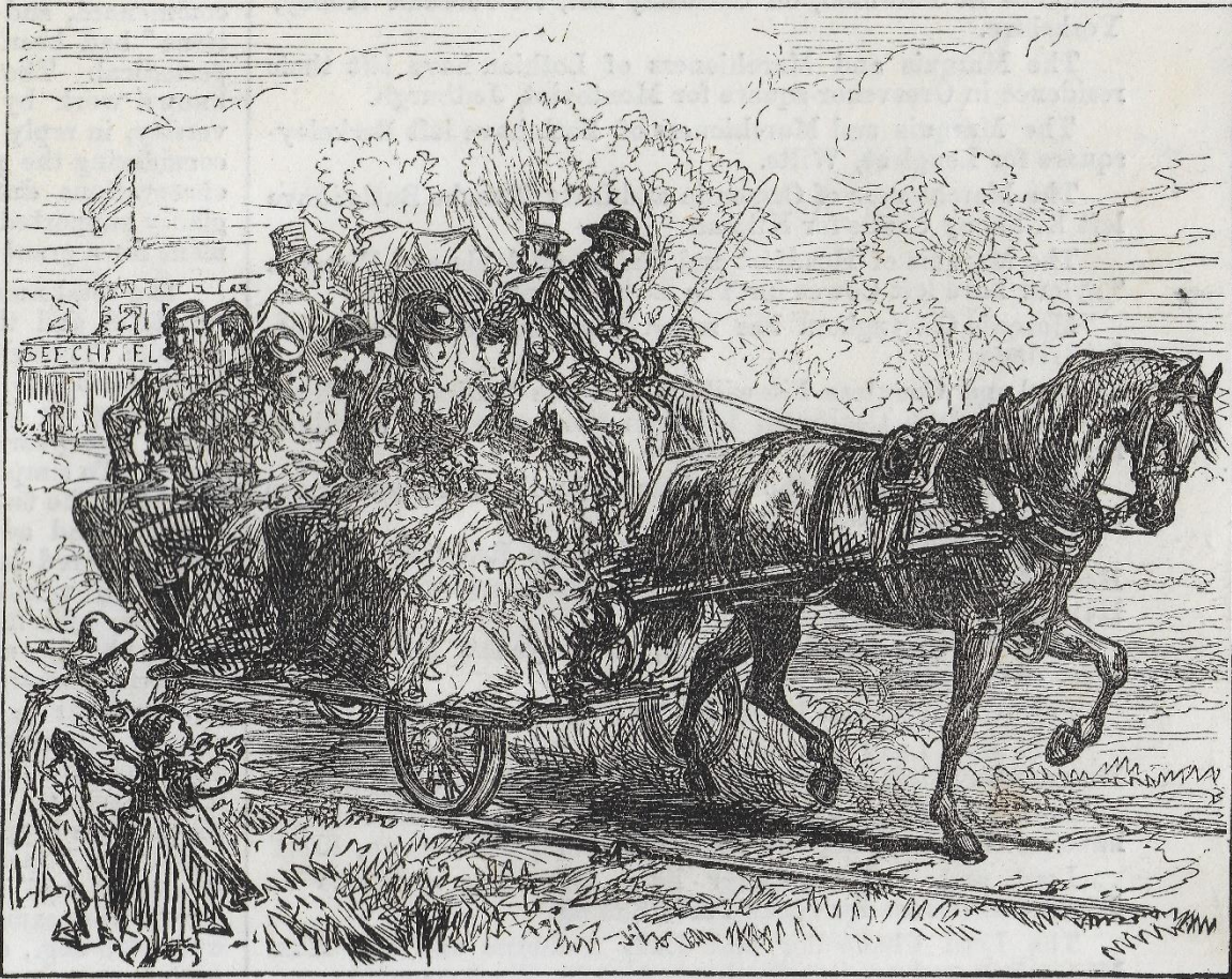
TRAM CAR FROM THE ROCK TO THE 1ST DIVISION.
