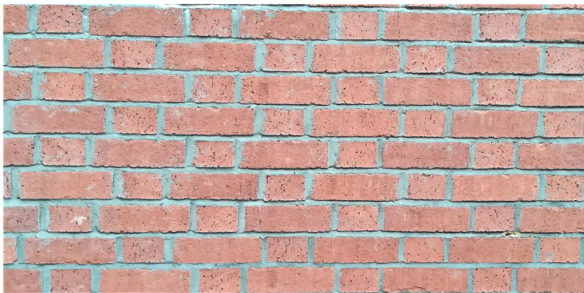
Figure 3.7 Flemish bond on Project A (photo taken by Orsolya Bokor in 2018)
