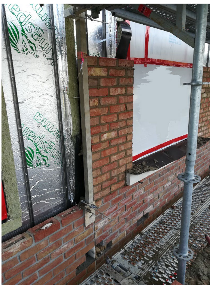
Figure 4.3 Profile and line (Photo taken by Orsolya Bokor in 2019)
