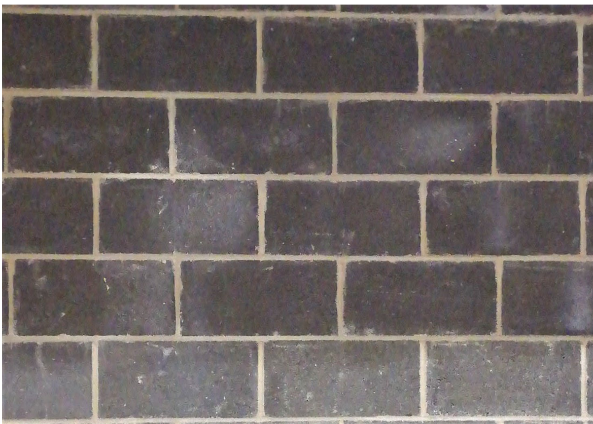
Figure 3.8. Blockwork on Project B (photo taken by Orsolya Bokor in 2019)
