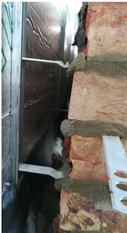
Figure 4.5 Ties (Photo taken by Orsolya Bokor in 2019)
