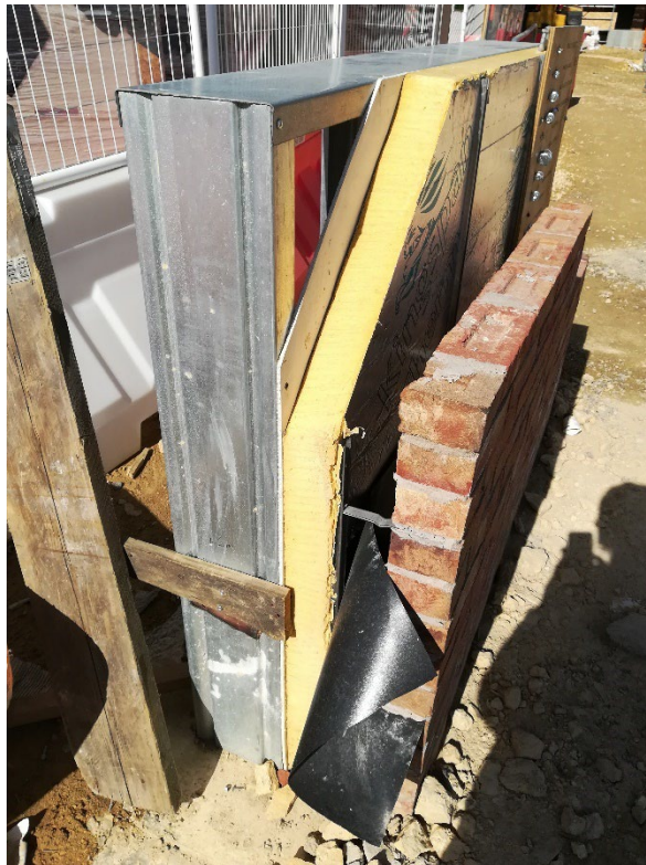
Figure 4.1 Cavity wall construction (Photo taken by Orsolya Bokor in 2019)
