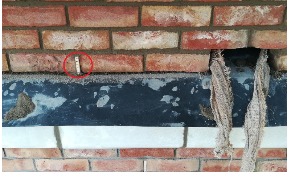
Figure 4.4 Hessian, weep, damp proof course (Photo taken by Orsolya Bokor in 2019)
