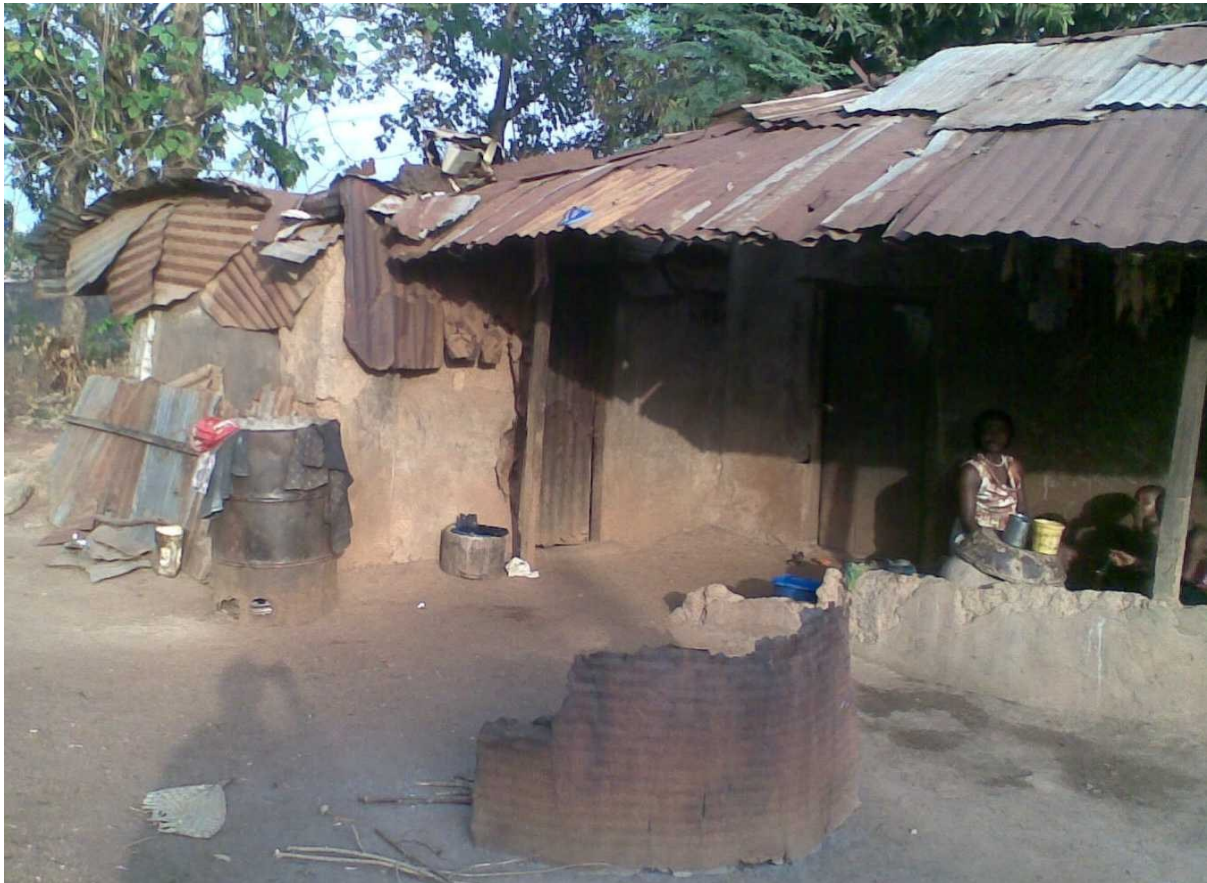
Figure 3: House with Rendered Clay Block Walls
