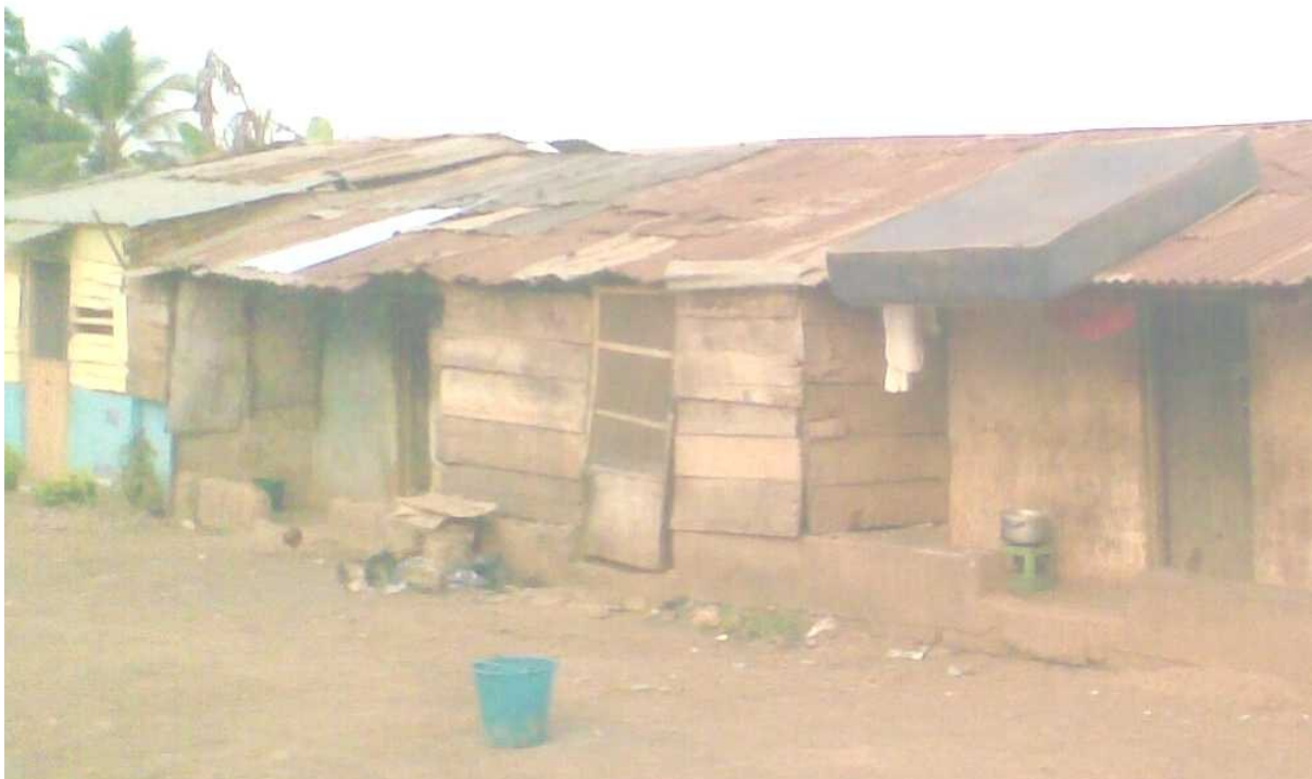
Figure 4: Houses with Reclaimed Timber Boards as Walls
