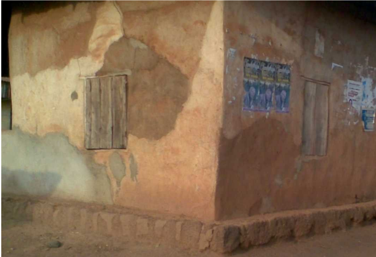
Figure 5: House with Timber Boards over Openings
