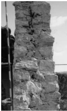
Figure 1 Double leaf wall
