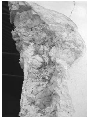
Figure 3 Only some spots were injected in the case of this wall with a very low percentage of voids.
