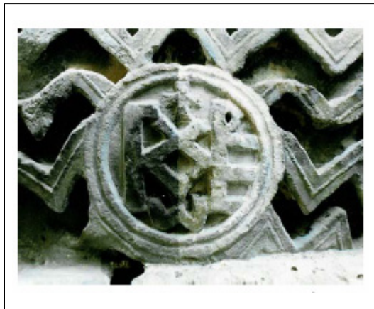
Figure 7. A laser cleaned section from the outdoor decoration of the 12 th century church of Panaghia Kapnikarea in the historical centre of Athens (Marakis, 2000) [62]. The application was carried out with the 3rd harmonic of the Nd:YAG laser (355 nm) using consecutive pulses at 0.4 and 0.5 J/cm 2 .
