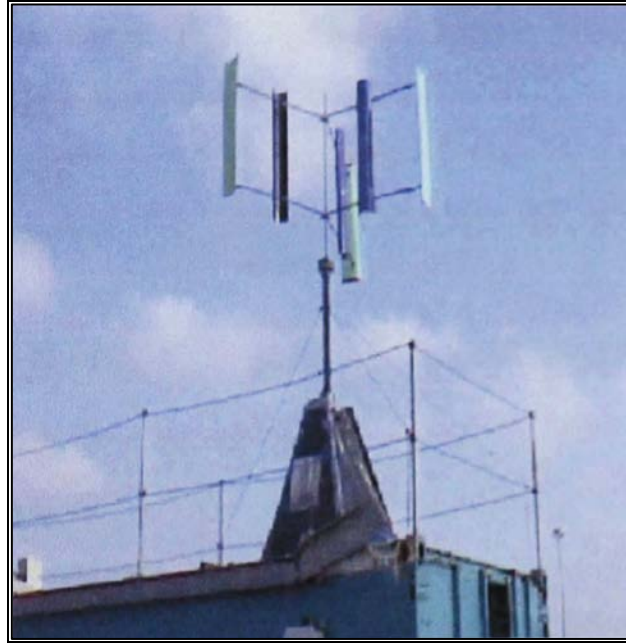
Fig. 6.29 The SCT attached to D-rotor at 0.4 m radius of VAWTs
