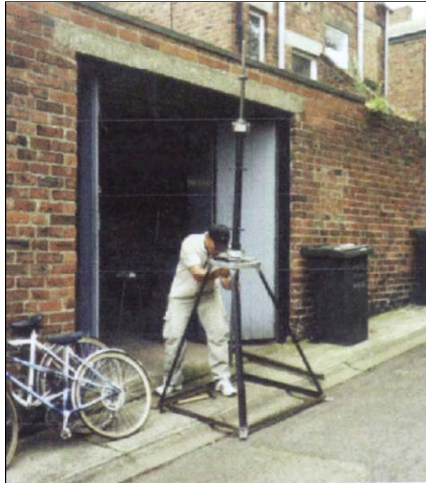
Fig. 6.5 Shaft and Shaft supporter on pre-assembling the wind machine
