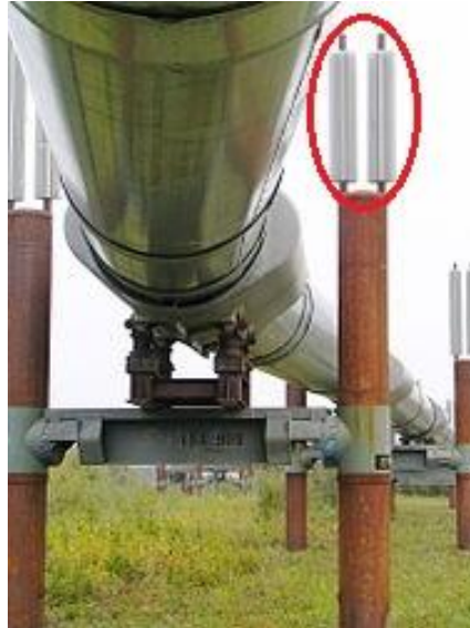
Figure 2- 4 Ammonia heat pipes used to stabilize the frozen soil under the Alaska pipeline. The finned ends of long heat pipe are seen at both sides of the pipeline at regular intervals
