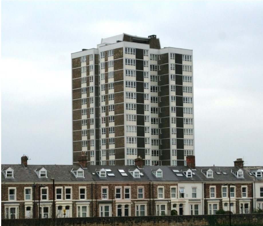
Figure 4 Photograph of King Charles Tower (17)
