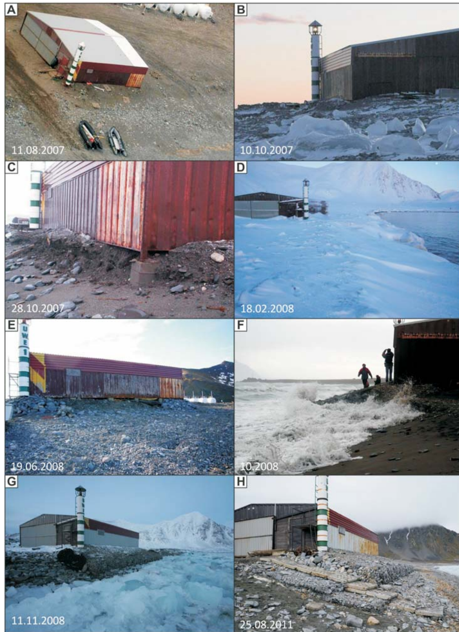
Fig. 8. The effects of coastal erosion processes in the area of harbour building of Polish Polar Station – “Banachówka” and methods of its protection. Photo: M. Błaszczyk archive (A–D, F), J. Kwaczyński (E, G), P. Zagórski (H).
