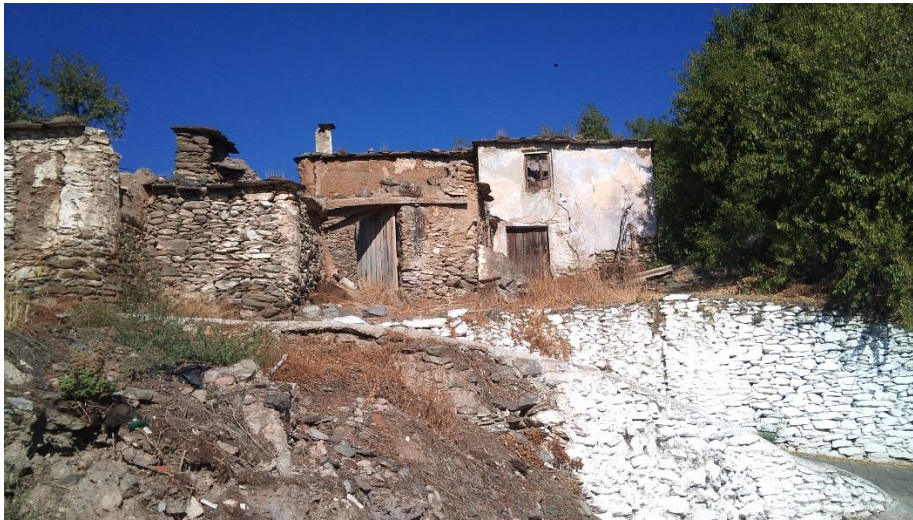
Figure 7: Ruined older property in Nechite, Válor municipio . (Source: Authors, Sept. 2012)
