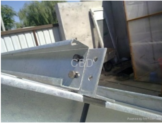
Figure 1: Application of roll-formed aluminium sections as flexural member, DIY Trade [2].
