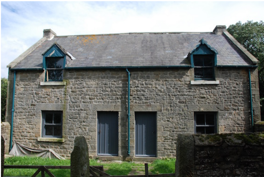
Figure 4.2: Orchard and Garden Cottages before refurbishment
