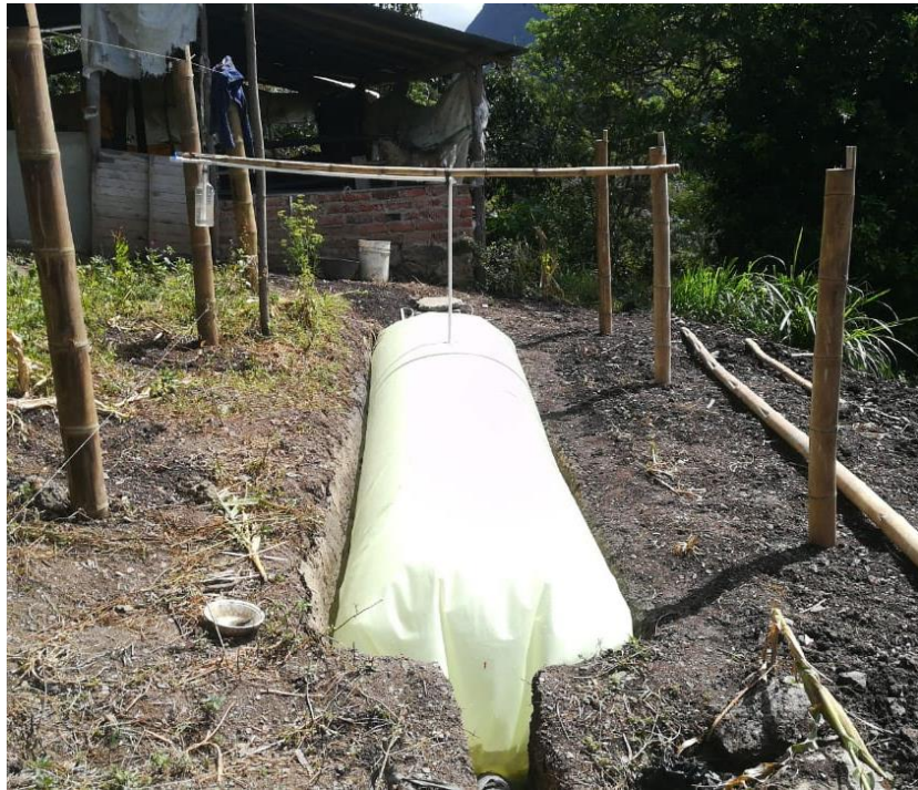
Figure 2. Household digesters installed by El Común.
