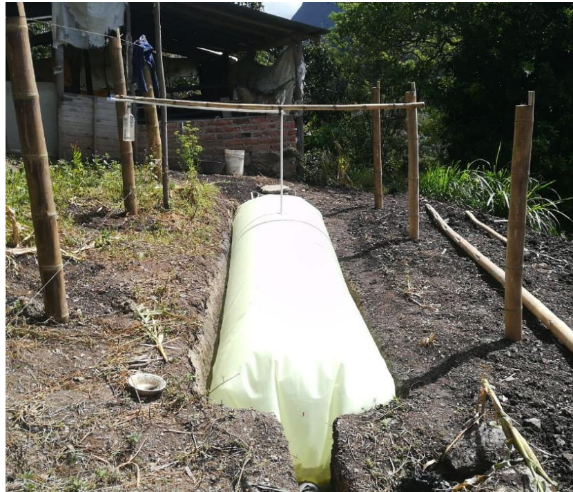
Figure 2. Household digesters installed by El Común. Image taken from the official website of El Común: www.elcomun.org
