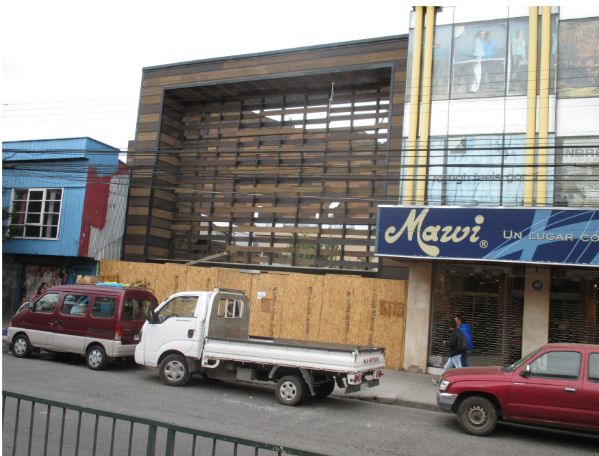
Figure 2. San Martín passage, still in construction (photo by author).
