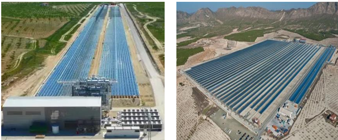
Figure 2.27: Novatec's linear Fresnel collector solar fields at the PE1 (Nova1) and PE2 (SuperNova) power stations (up to 520°C) [86]
