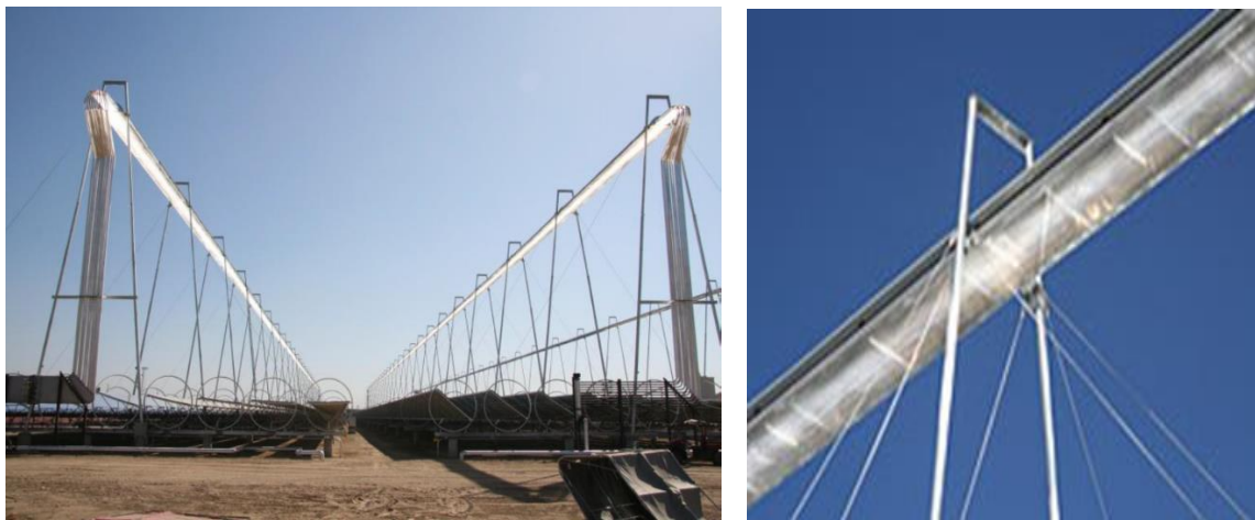
Figure 2.26: Areva Solar’s compact linear Fresnel reflectors at the Kimberlina power station (up to 482°C) in California with multiple tube receiver with simple trapezoidal secondary reflector [86]
