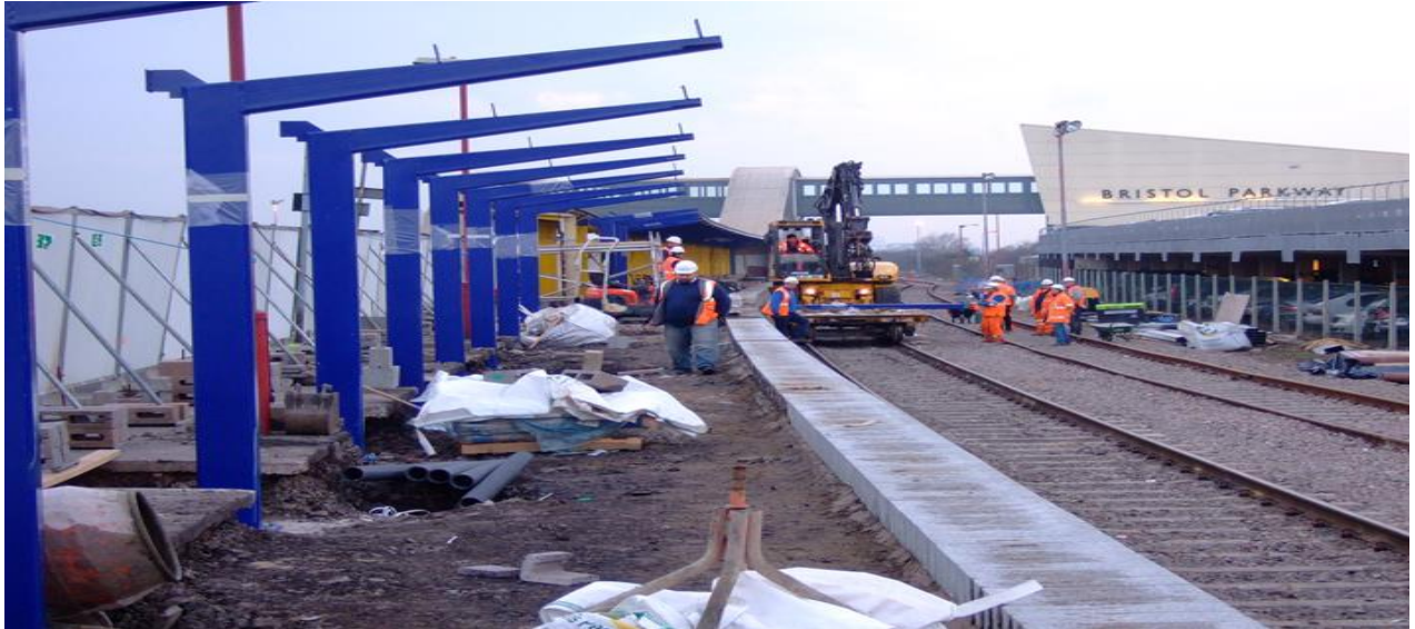
Fig-5.9 Showing the construction rail-station/platform in South of England (Railway, 2014)
