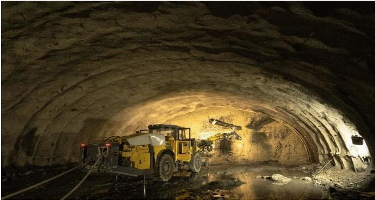
Fig 5.10 Showing the construction of tunnels/earthworks in South of England (Railway,2014)
