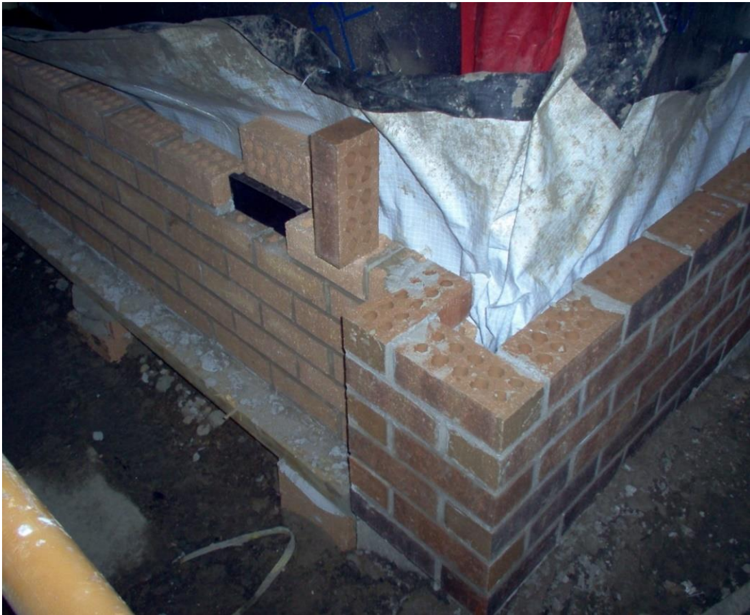
Figure 5.11: External cavity wall – pier (Photo M.3.1.).
