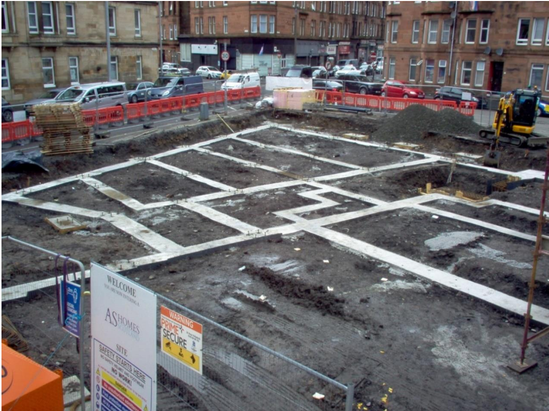
Figure 5.7: Holding down bolts after removal of formers (Photo C.3.7).
