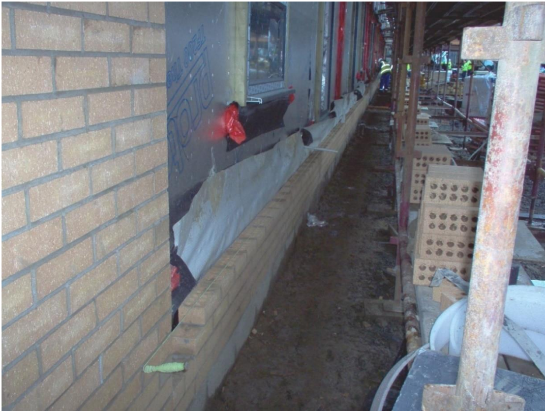
Figure 5.10: External skin of cavity wall (Photo M.2.1.).
