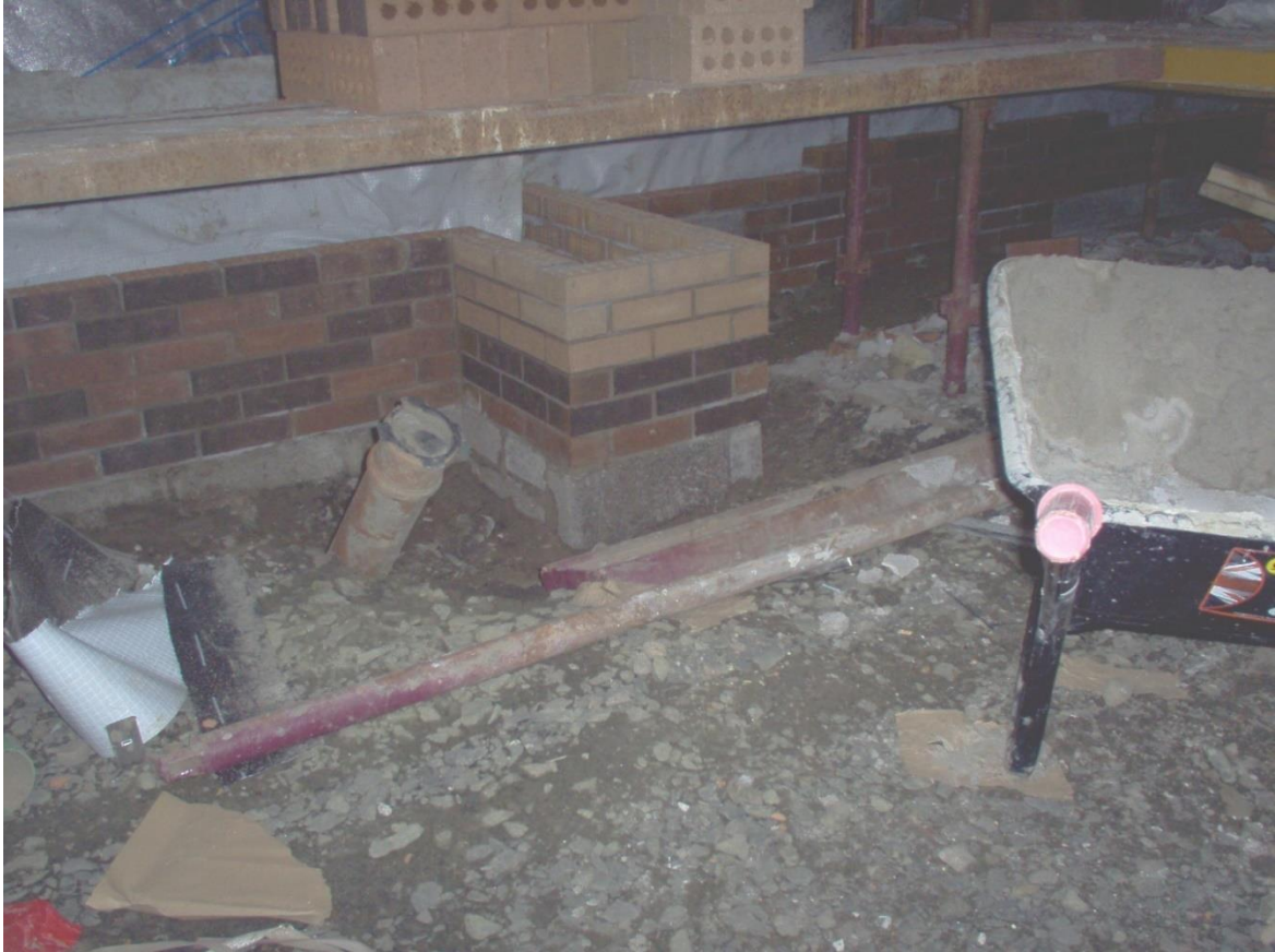
Figure 5.12: Pier at an entrance (Photo M.4.1.).
