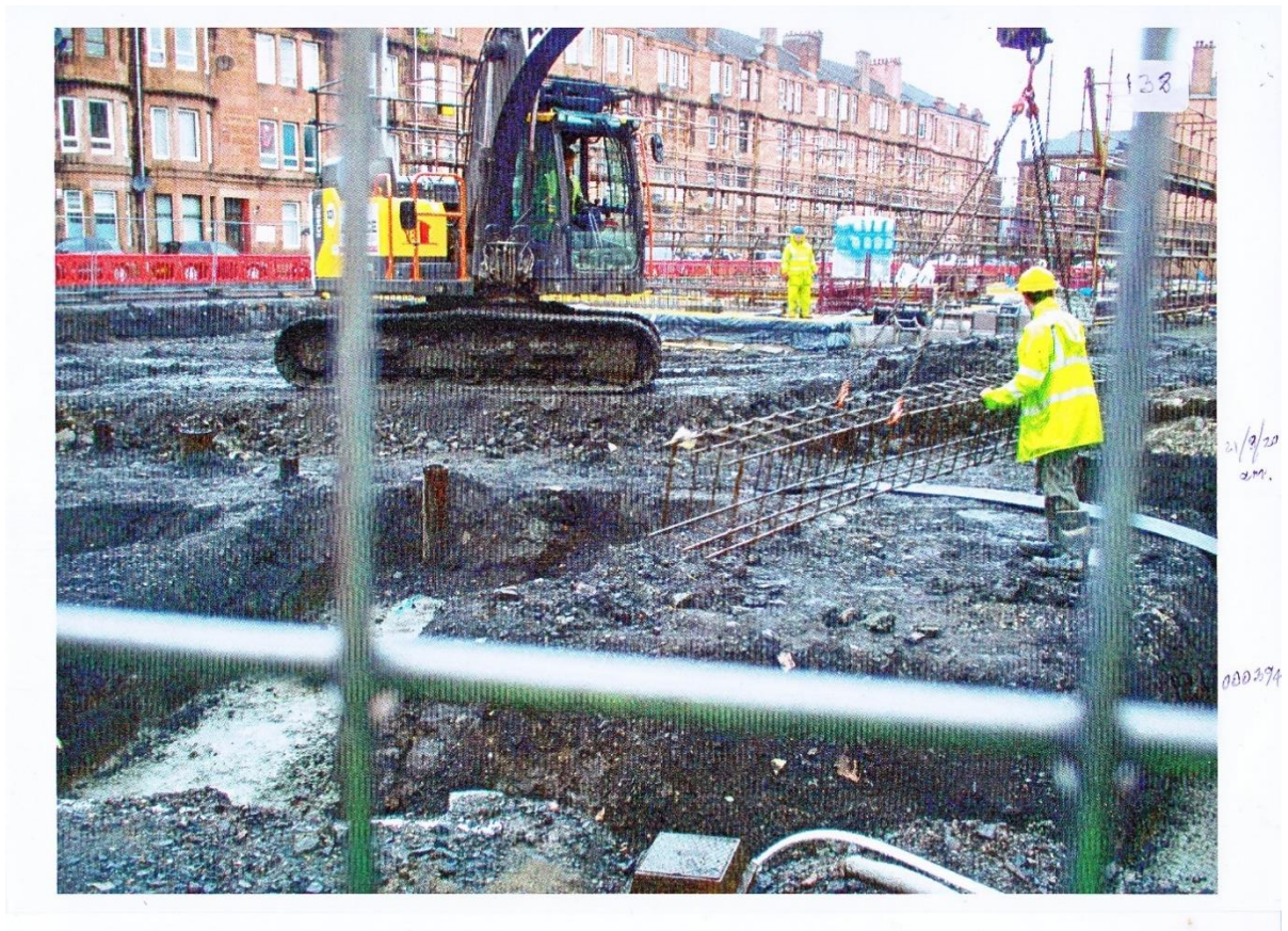
Figure 5.5: Transporting completed section of ground-beam cage (Photo C.1.5).
