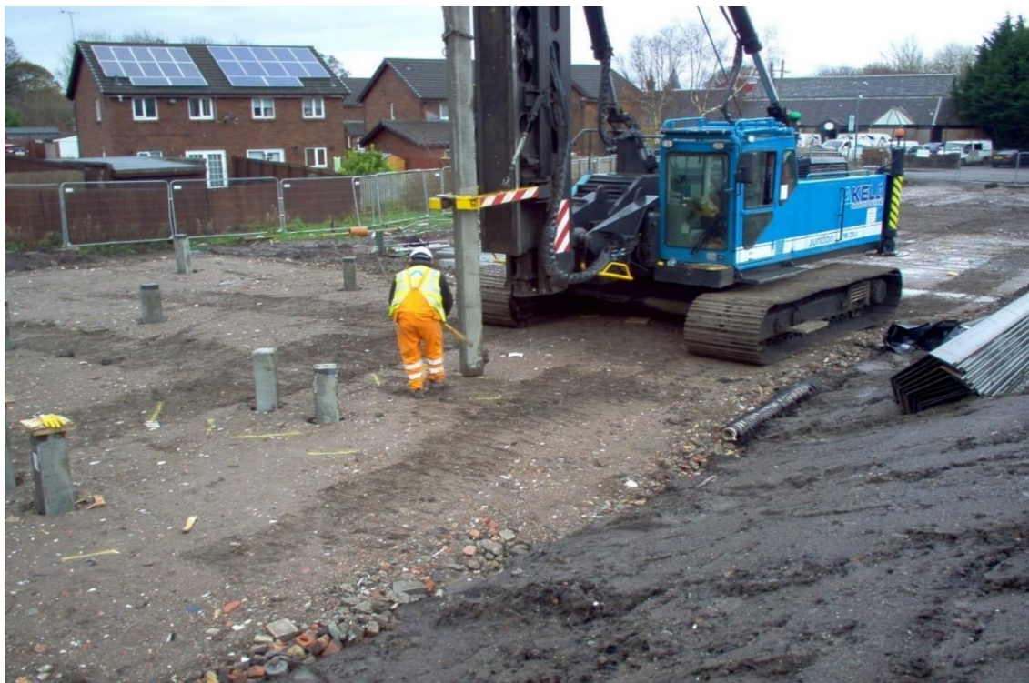
Figure 5.3: Pile being positioned (Photo E.3.3.).
