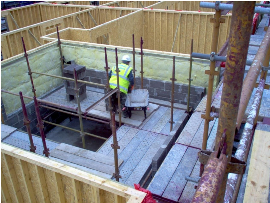
Figure 5.9: Blockwork in common parts stairwell (Photo M.1.5.).
