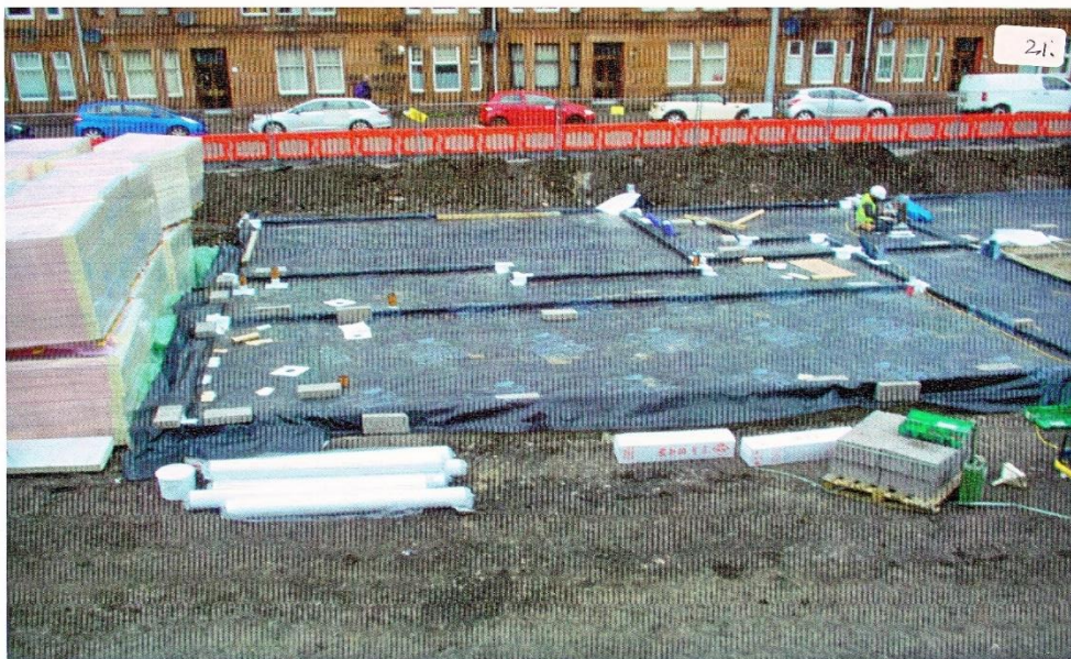
Figure 5.2: Laying gas proof membrane (Photo E.2.4).
