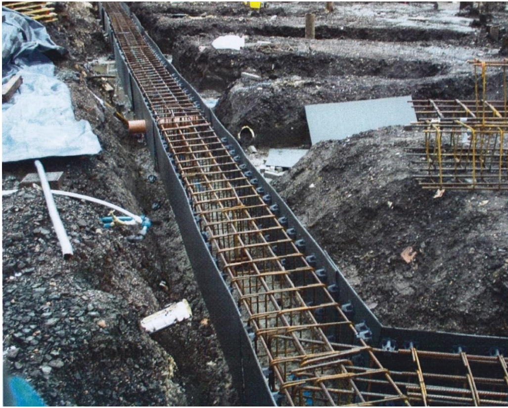
Figure 5.6: Shuttering to ground beam (Photo No C.2.1).
