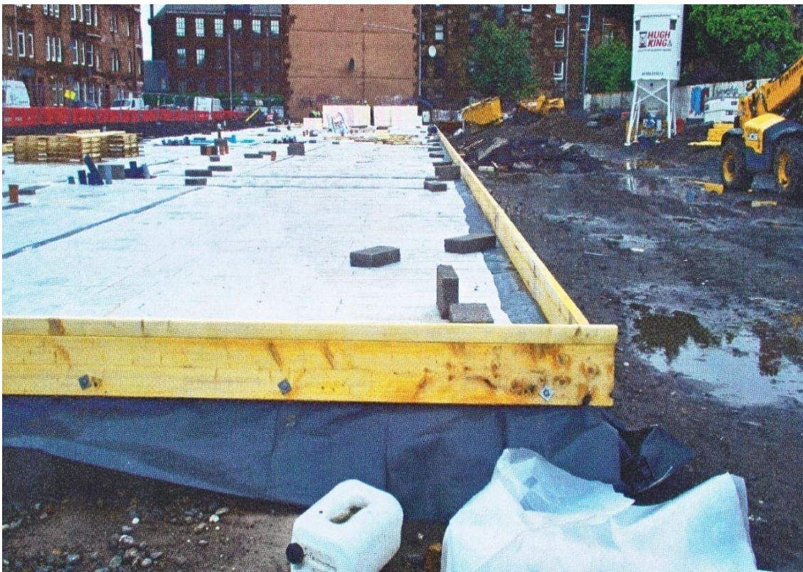
Figure 5.8: Shuttering edge of slab (Photo C.4.4.).
