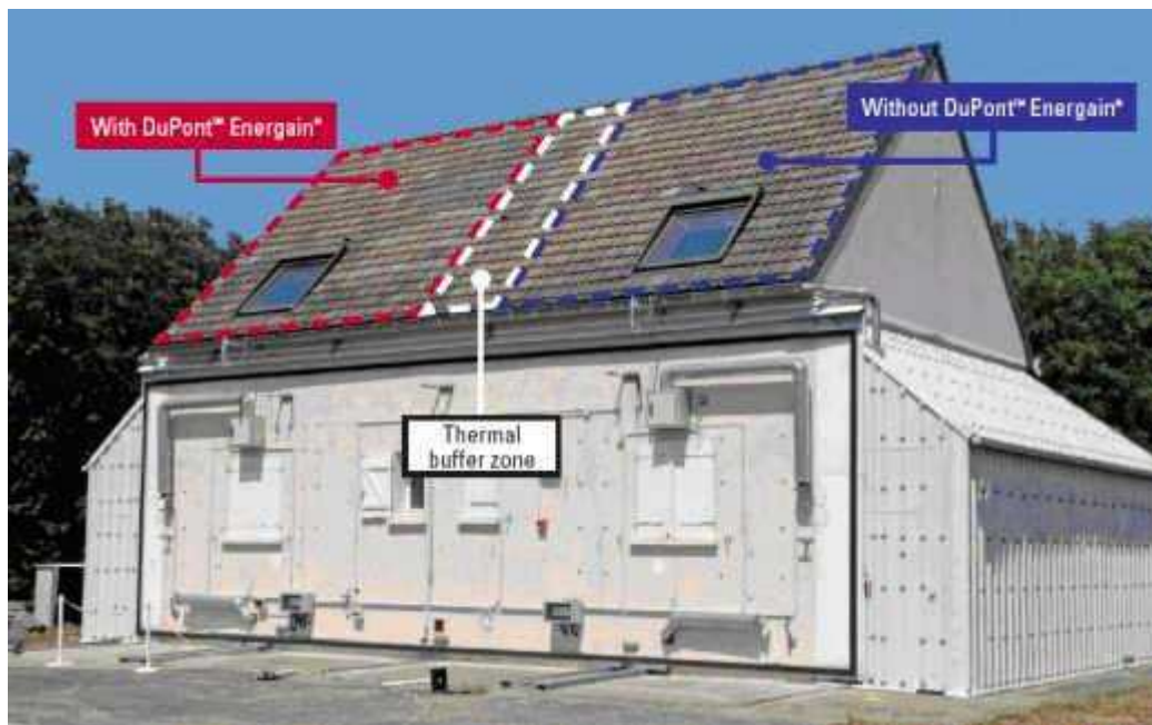
Figure 10: DuPont's test house in France (DuPont, 2008)
