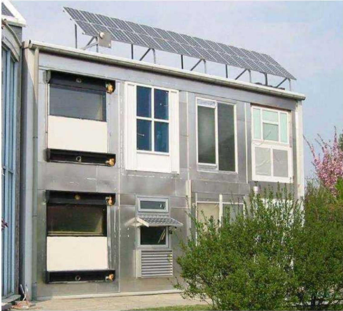
Figure 4: Fraunhofer ISE façade testing facility. The test offices are the two rooms at the left hand end of the building (Schossig et al, 2005).
