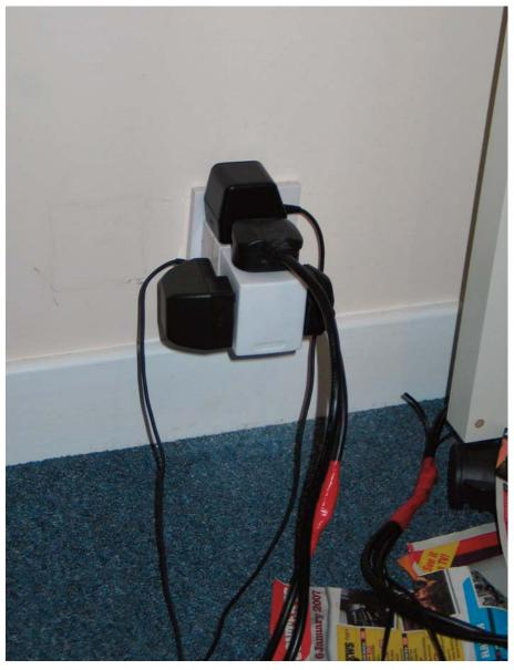
Plate 4 Demonstration of High Risk Wiring
